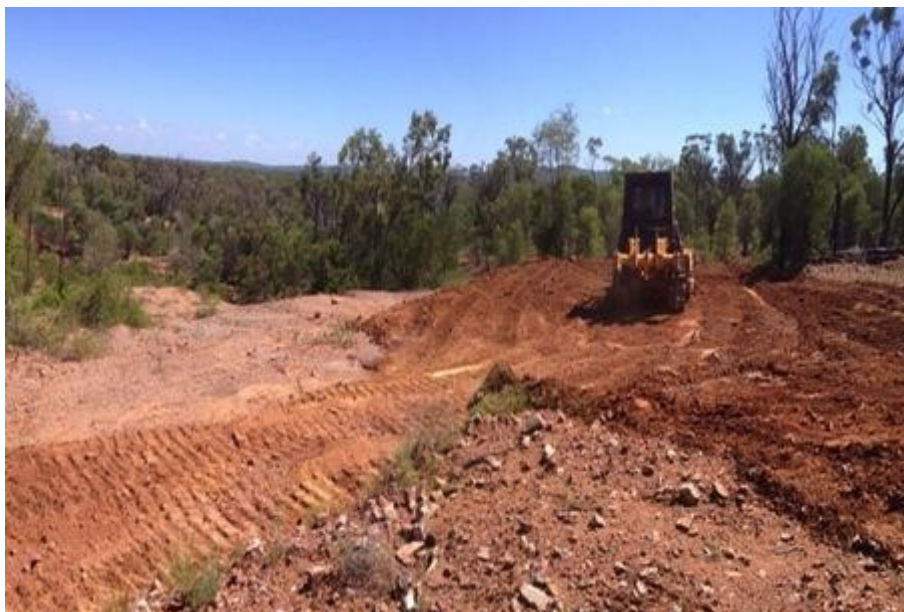
IMAGE 1. Site remediation - Pyramid project
